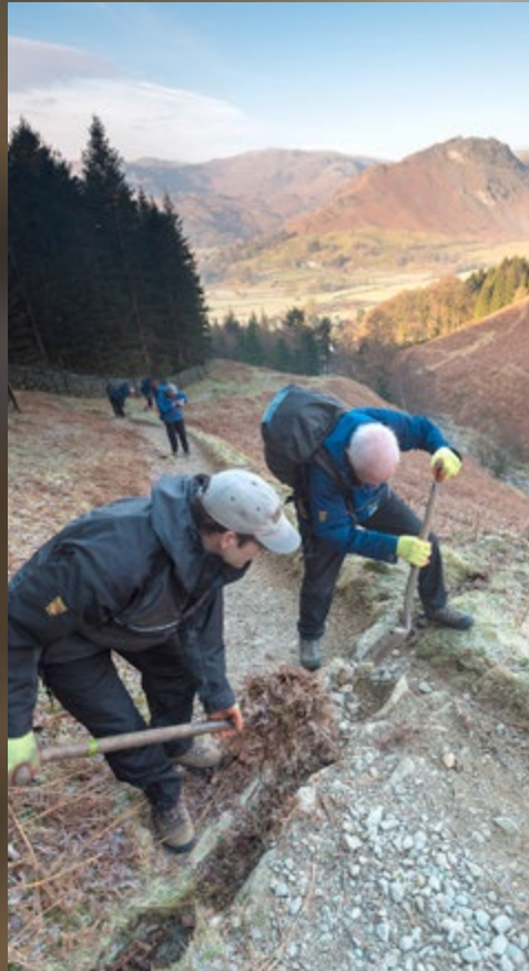
Rangers and volunteers helping to clear pathway drainage on the fells above Grasmere, Cumbria
