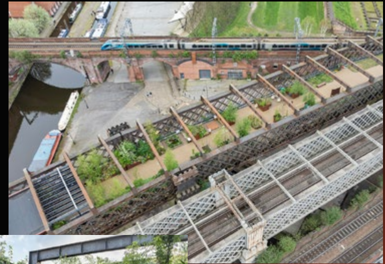
Aerial view of Castlefield Viaduct, Manchester, Greater Manchester
