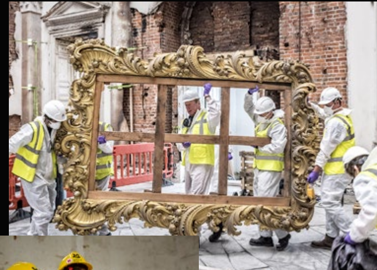
Conservationists working on the Clandon Park restoration project, Clandon Park, Surrey
